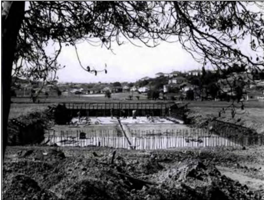
Figure 2.16 Photograph taken during construction of the Pool. The surrounding fill and excavation is visible.
