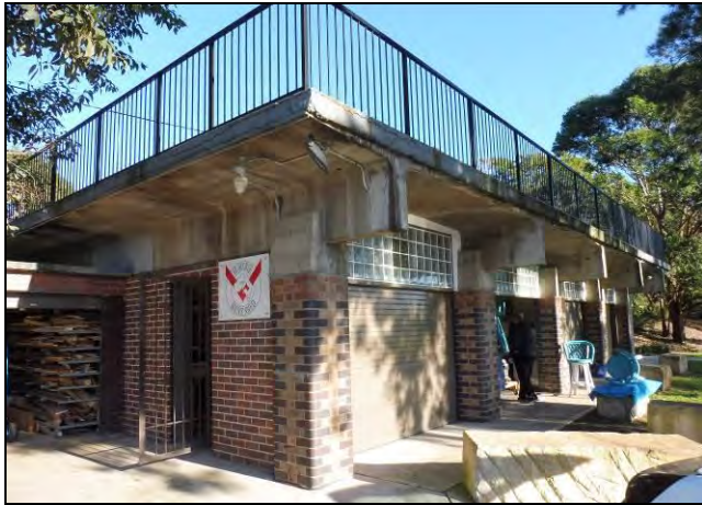
Figure 3.34 The Men's Shed retains part of the early, Inter-war period pavilion (brick columns) to which brick and glass block infill and additions and a concrete structure (roof deck) have been added.
