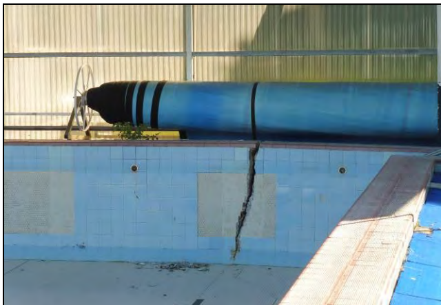
Figure 3.64 A large crack is located near the north eastern corner of the 50m pool.
