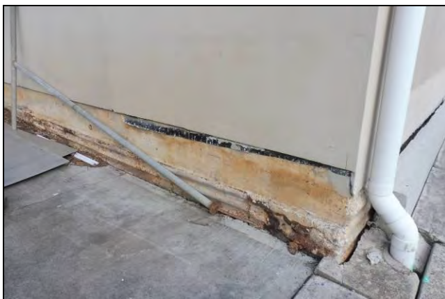
Figure 3.44 Some cracking and movement/subsidence is visible at the base of the central bay. A concrete step has also been added to the base of the front façade. Some corrosion and failure of the footing is also evident along the northern side.
